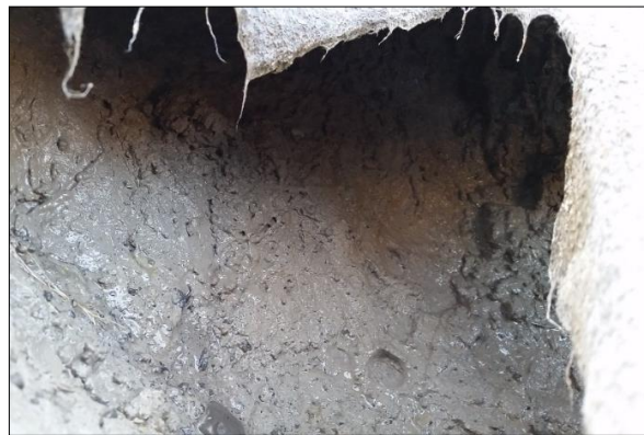
Photo 3. Yielded geotextile over wet grade
