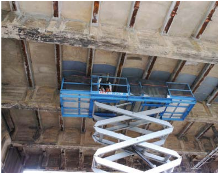
Installing FRP on the underside of concrete arches off scissor lift
