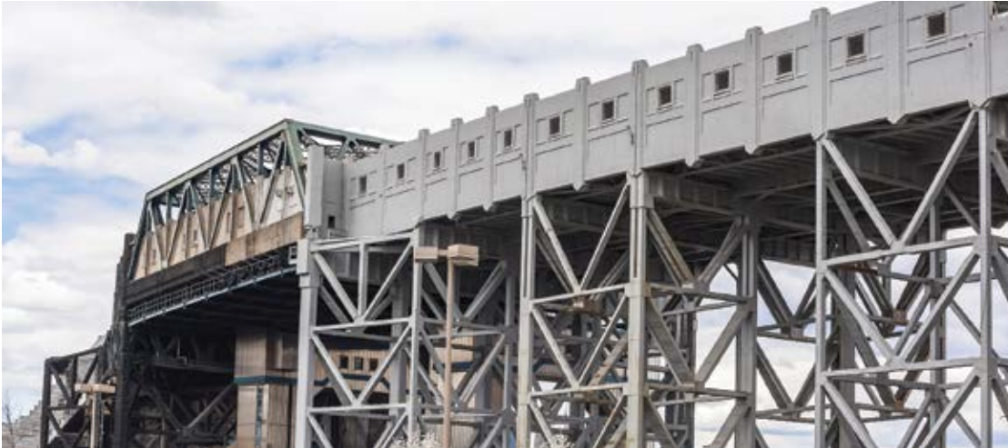
Culver Line Viaduct after concrete repairs
