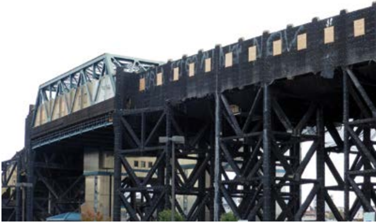
Culver Line Viaduct prior to concrete repairs
