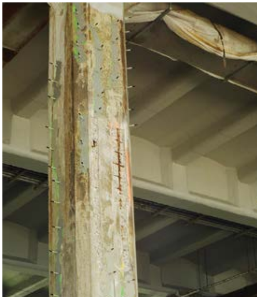
Epoxy injection of cracks on a column
