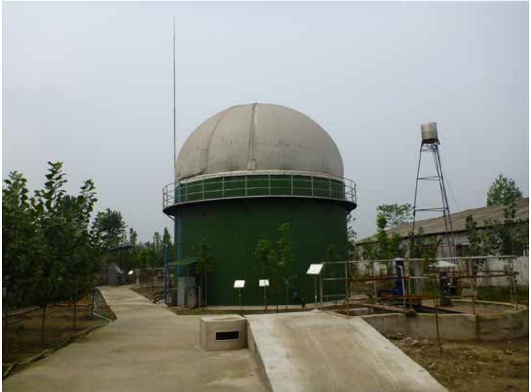
*400 cubic meter biogas digester with flexible storage membrane on top.*
