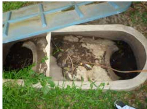
*Fibreglass modular system installed (looking from above) showing inflow to the left, outflow to the right and gas line in the middle.*
