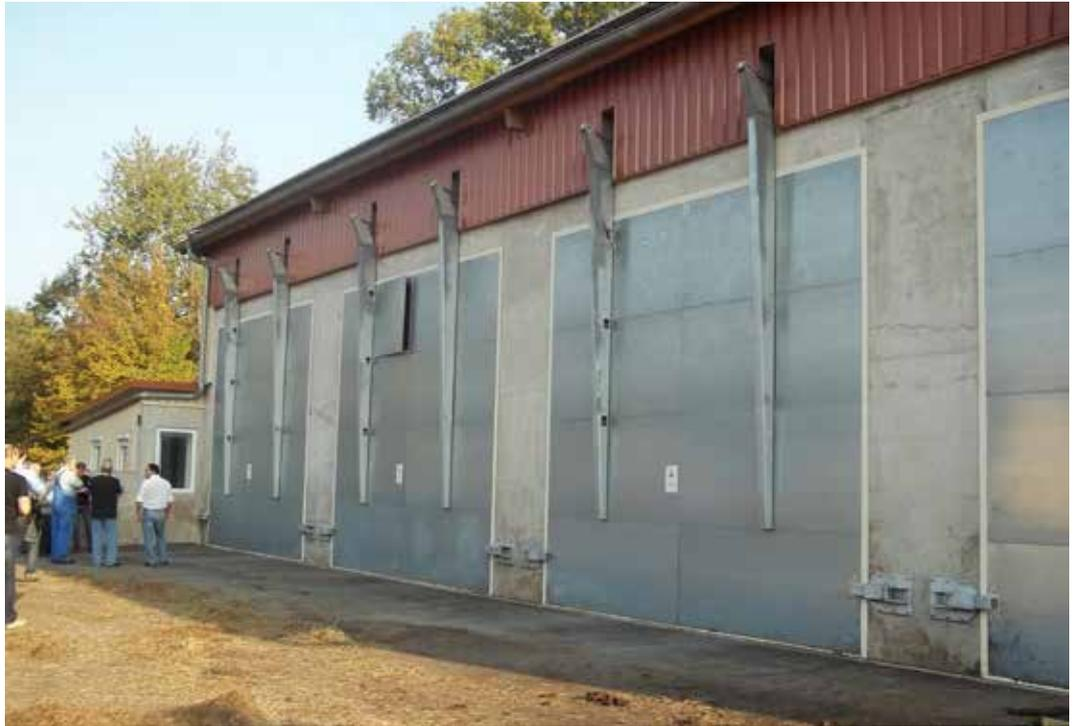
Garage digester showing individual 'garage' chamber doors. These doors are hinged at the top.
