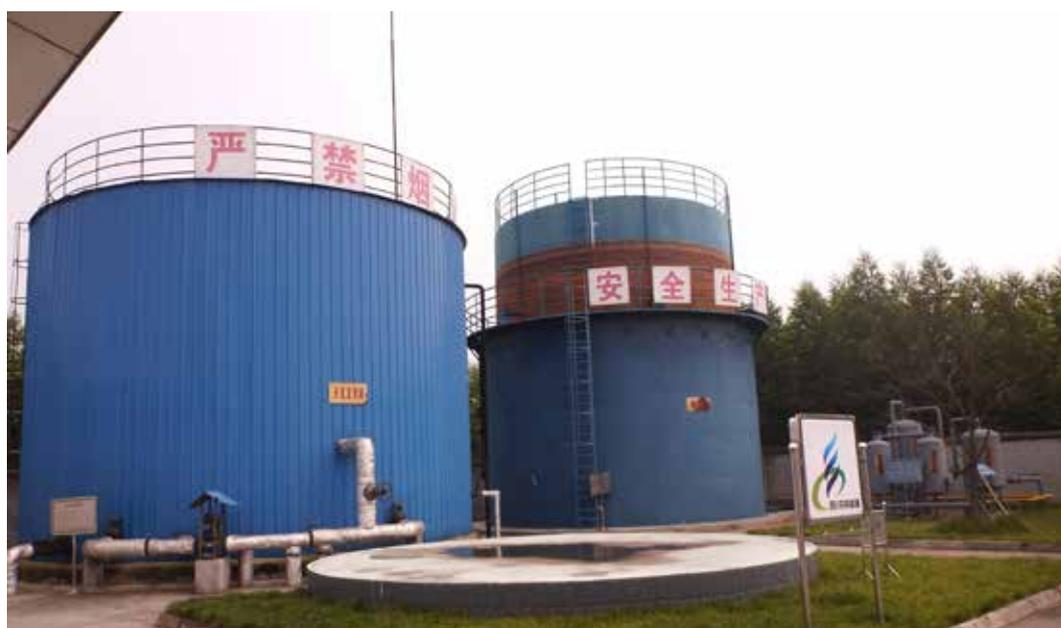
*Biogas digester to the left and a floating tank storage gas storage vessel to the right. This system enables the gas to be pressurised for distribution.*
