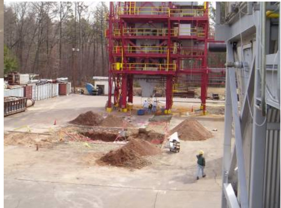
South View of BSF - Excavation For Oxygen Supply Foundation
