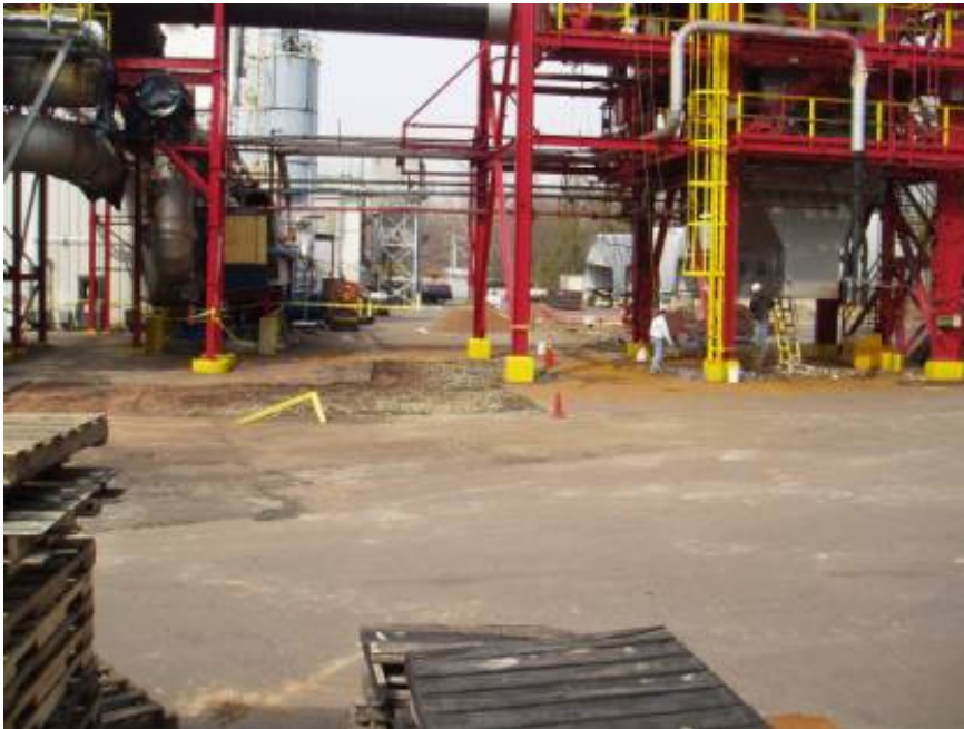
North View of BSF- Excavation For Fabric Filter Foundation
