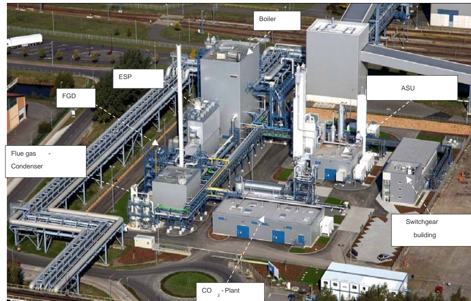
Vattenfall AB – 30 MWt Oxy Plant at Schwarze Pumpe Station
