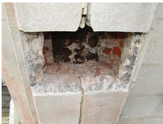
Fig. 4: Brick infill around steel column
