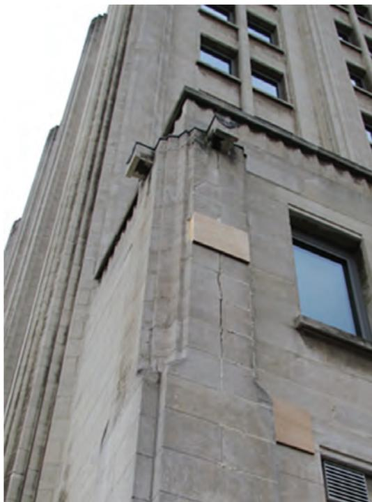
Fig. 3: Vertical cracking at column
