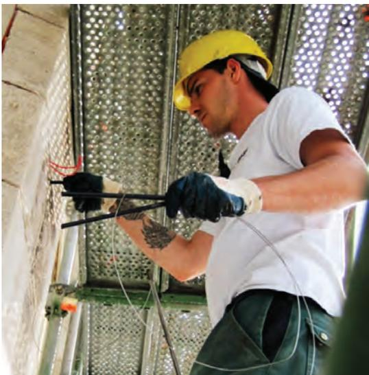
Fig. 14: Conductive titanium dioxide ICCP anode placement
