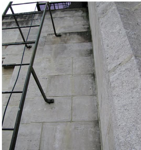
Fig. 16: Anodes and wires concealed
