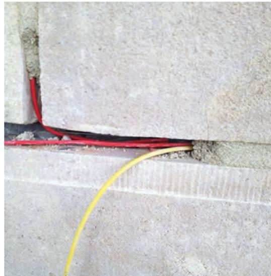
Fig. 15: Wiring concealed in the mortar joint
