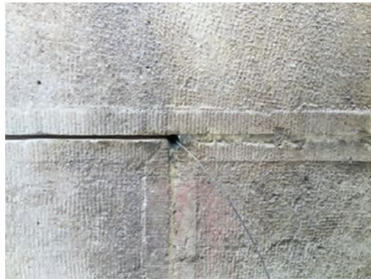
Fig. 7: Discrete anode in masonry joint
