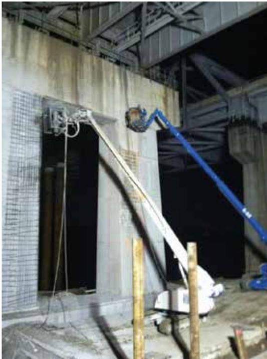
Fig. 3: Operator in manlift observing the hydrodemolition
