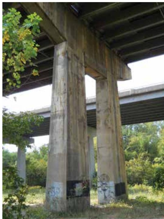
Fig. 2: Substructure pier in need of repair
