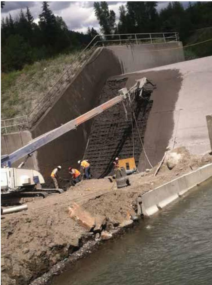
Fig. 7: Hydrodemolition unit removing concrete from the spillway face
