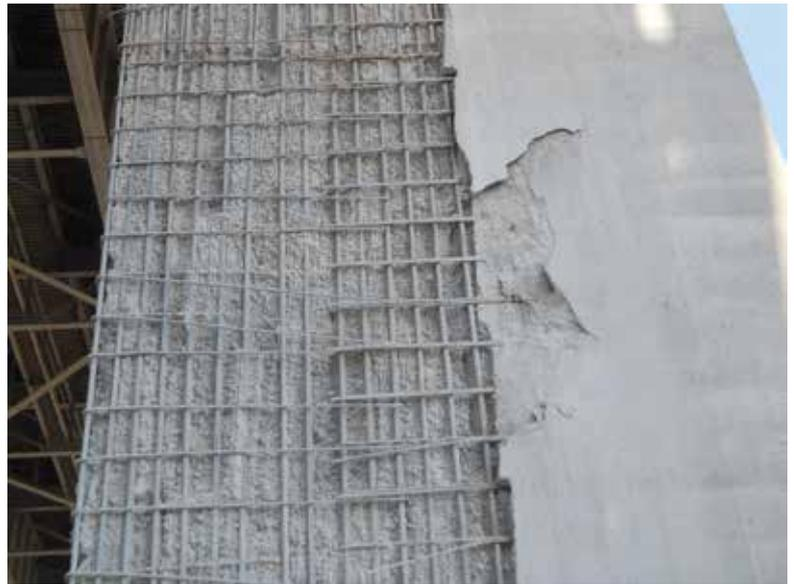
Fig. 4: Removal area adjacent to delaminated concrete
