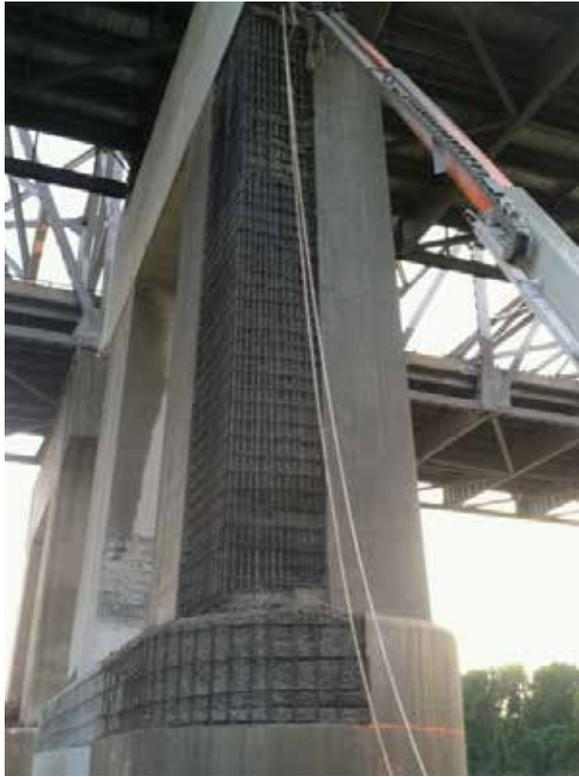
Fig. 5: Full height concrete removal on 25% of the pier
