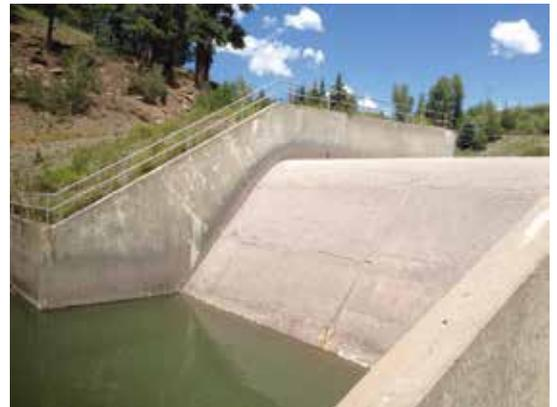
Fig. 6: Blanco Diversion Dam Ogee Spillway removal area adjacent to delaminated concrete
