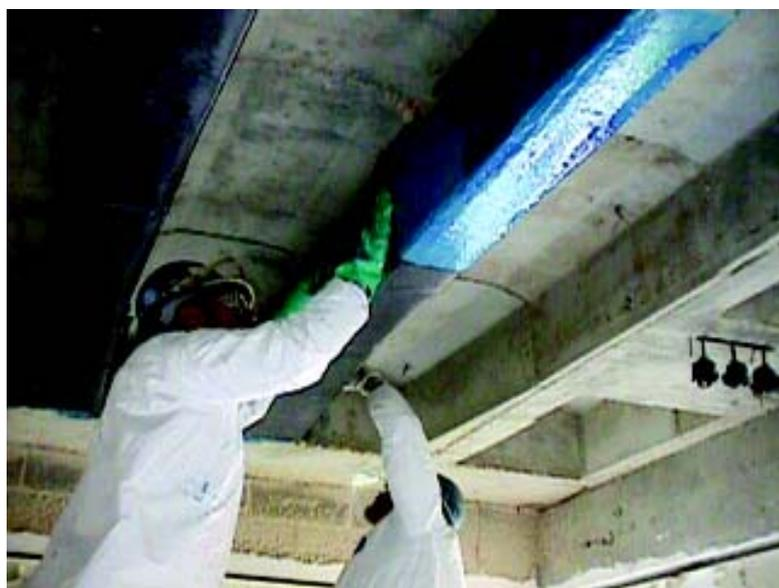
Figure 1: Application of FRP sheet on one-way joist
