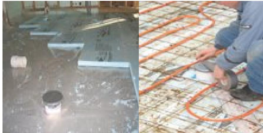
Figure 8. (a) Extruded polystyrene insulation layer is placed on the concrete slab (left side) and (b) the reinforcing wires together with the tubing of the floor heating system are placed (right side).
