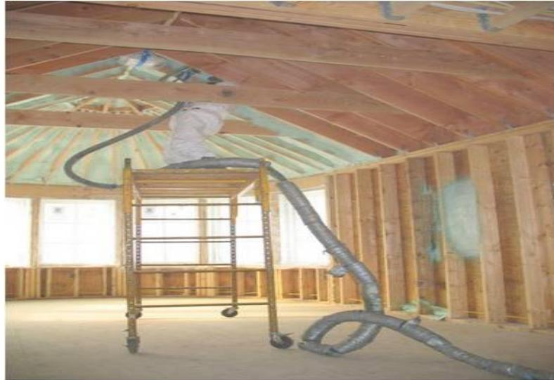
Figure 7 Room with walls and ceiling filled with the sprayed polyurethane foam
