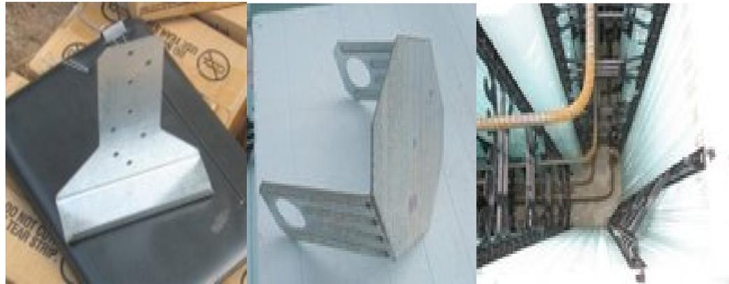
Figure 2: The selected ICF system provides brackets for hanging the joists (left) support plates (center) and bracing for corners (right side).
