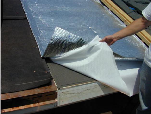
**Figure 4. Residential Attic Containing Dynamic Reflective Insulation**
