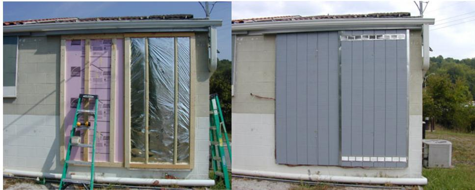
**Figure 6. Experimental wall containing PCM-enhanced reflective insulation.**
