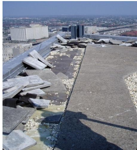
Figure 4: Type C low parapet (less than 36 inches in height) often creates a false sense of protection along the roof edge.
