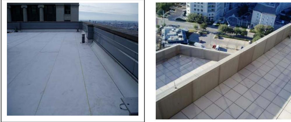
Figure 5: Type D full 42 inch high parapet offering the best protection against wind forces as well as user safety.
