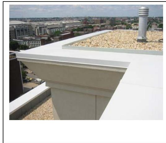
Figure 7: Air and thermal barrier continuity demands scrutiny when roof appendages and wall edge extensions are incorporated into the design.
