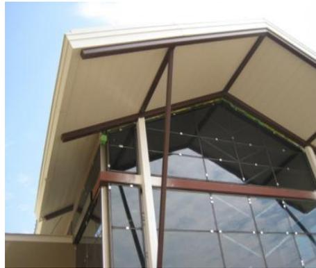
Figure 2: The Type A sloped roof overhang at top of wall poses difficulty (red highlights) in maintaining air and thermal barrier provisions. Roof drainage must also be suitably designed along the roof edge.
