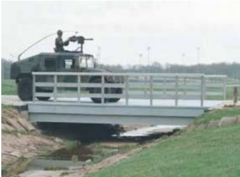
Figure 4 - RPL pedestrian and vehicular bridge at Fort Leonard Wood, Missouri.
