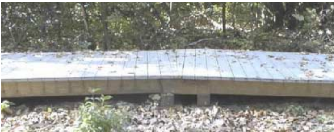
Figure 3 -Wooden substructure for Kelleys Island RPL boardwalk.
