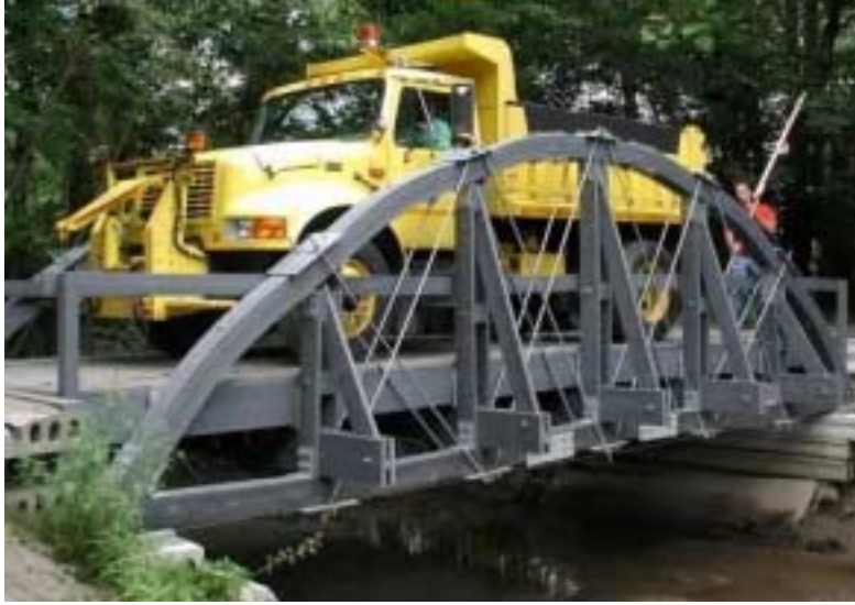
Figure 7 - RPL arch truss bridge near Albany, New York.
