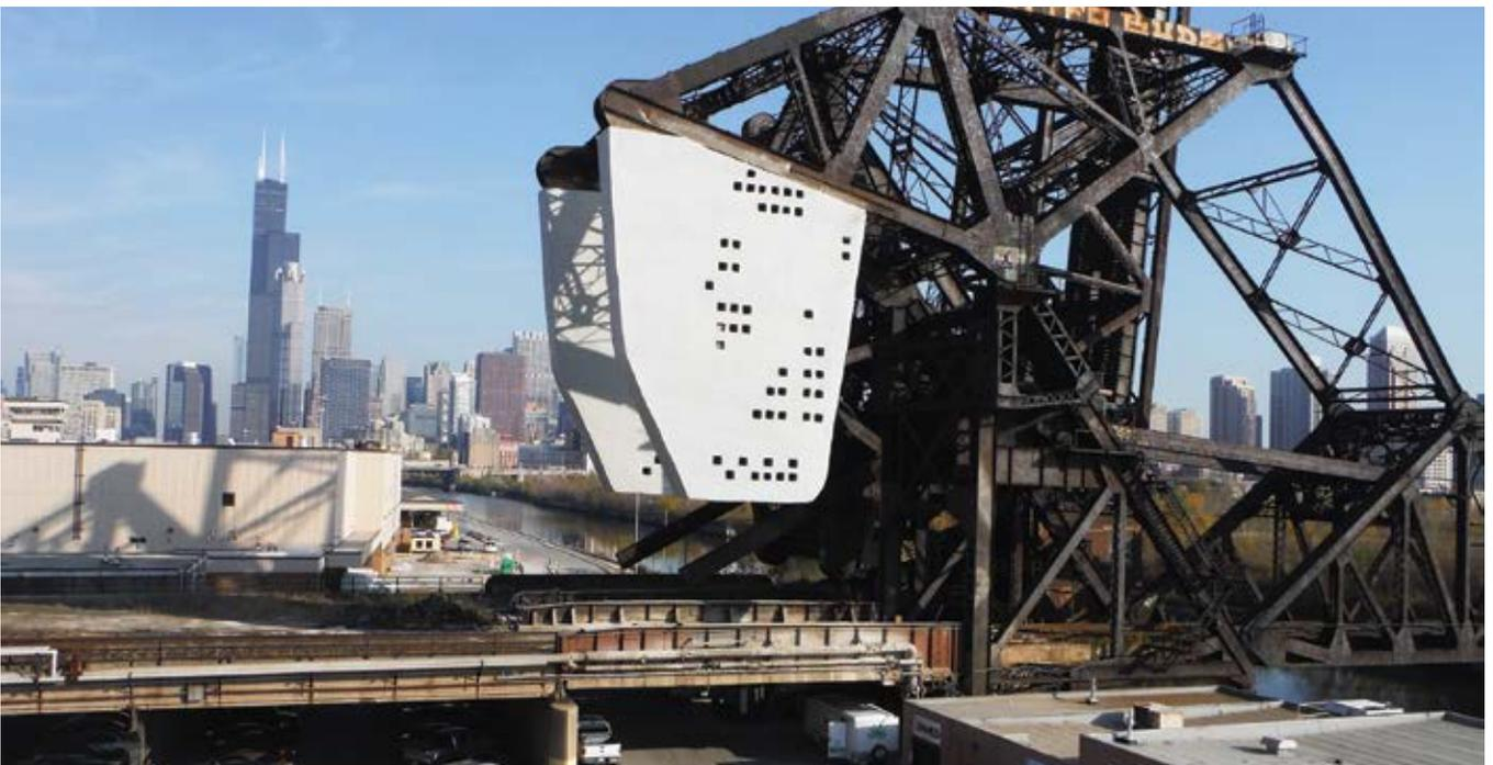
Fig. 12: The repaired counterweights with surface-applied FRP and a light gray acrylic topcoat
