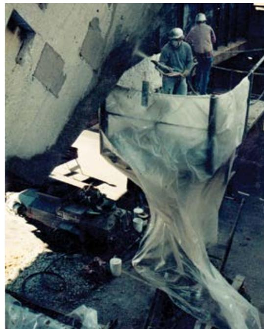
*Fig. 10: Wet-mix shotcrete was selected for the repair material*
