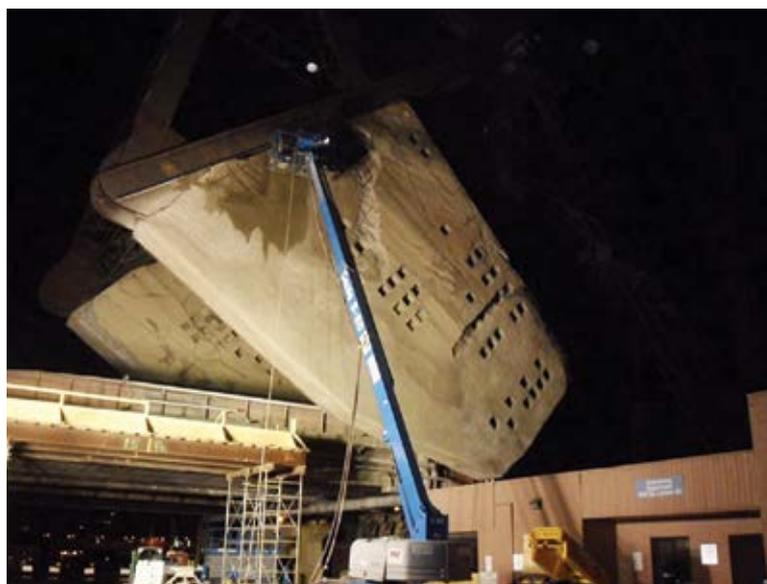
*Fig. 9: The bridge was raised at night to allow counterweight access by boom lift*
