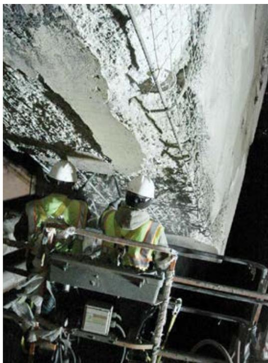
*Fig. 8: Concrete removal was limited to 3 yd<sup>3</sup> (2.3 m<sup>3</sup>) to maintain balance during repairs*
