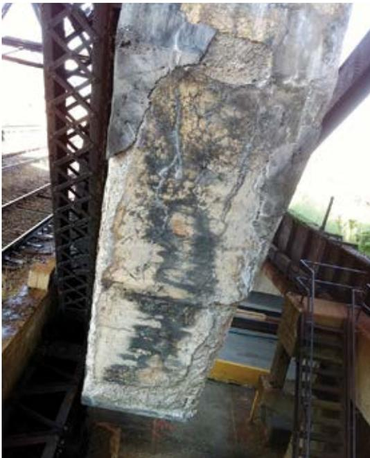
Fig. 6: Condition of the winged concrete counterweight
