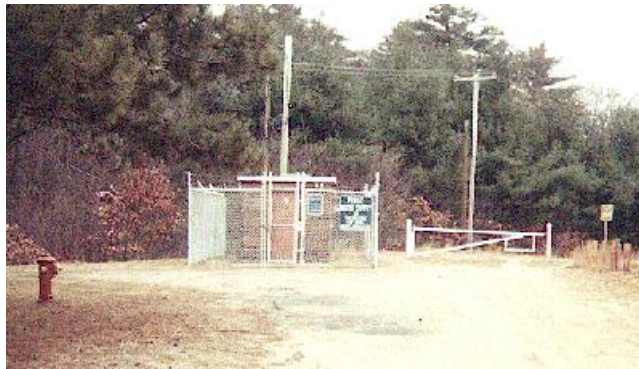
MUNICIPAL WATER SUPPLY PUMP HOUSE
