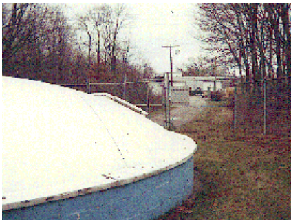
A water supply treatment plant and pump house with a public works garage 300 feet away
